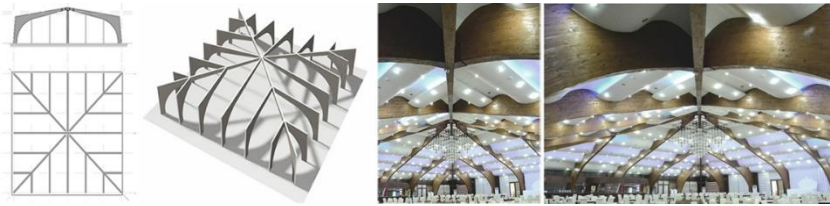
Figure 14. Large span glue laminated timber structure, Pejë
