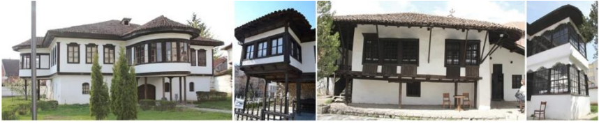
Figure 2. Combined structure house Kosovo
