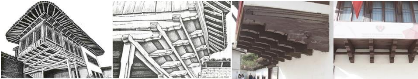
Figure 6. Wooden jetty drawings on the left (Doli, 2001) , the rest by the author
