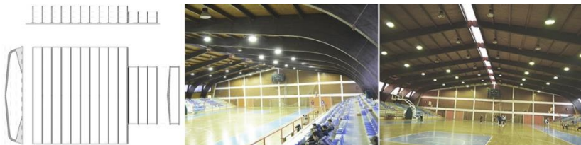
Figure 15. Large span glulam timber structure, Vushtrri
