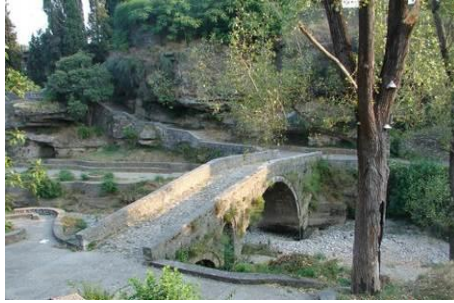
Figure 29. Bridge on the Ribnica river, Podgorica, Montenegro (16th century) (Photo: http://www.panoramio.com/photo/13857943 )
