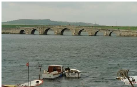
Figure 19. Sultan Suleiman the bridge, Büyükçekmece, Turkey (1568)
