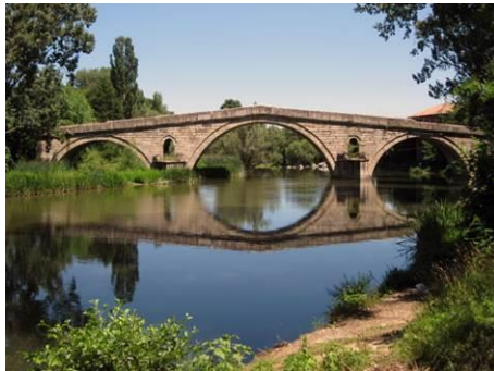
Figure 22. Kadin Bridge on the Struga river Nevestino, Bulgaria (1470)
