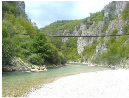
Figure 03. Suspension Bridge on the Neretva River (Photo: http://www.panoramio.com/photo/5138547 )
