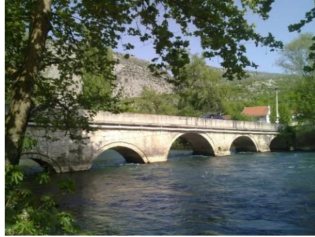
Figure 11. Karadžobeg bridge on the river Buna in Blagaj (Photo: Professor A. Hadrović, PhD, 01.05.2013.)
