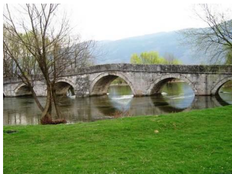
Figure 07. Bridge at Plandište ("Roman Bridge"), Ilidza near Sarajevo
