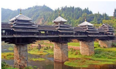
Figure 05. Chengyang Bridge, China (1912)
